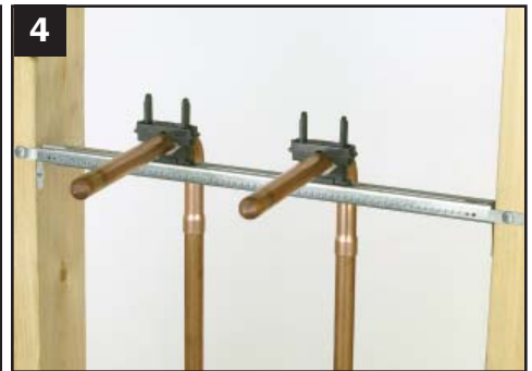
4 Place tube inside clamps and cinch the bridge down evenly over posts to secure.
