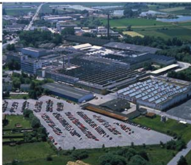
Stiebel Eltron's plant in Holzminden, Germany.
