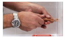
**8.** Insert repair adapter into tube in wall and wipe away excess epoxy on exterior of tube.
