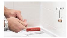
**2.** Remove any old fittings with hacksaw, making sure to leave at least a 1-1/4" length of copper tube exiting the wall.
