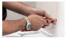
**4.** Dry fit repair adapter to make sure it fully slips into copper tube in wall.
