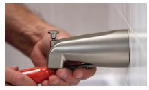
**5.** Tighten the screw to secure the SmartSpout snug to the wall. Do NOT over tighten as the wall could become damaged.
