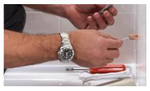
**7.** Then apply epoxy completely to inside of tube in wall.
