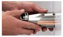
**2.** Mark the copper stub out even with the hash mark on the underside of the SmartSpout and cut off excess pipe.
