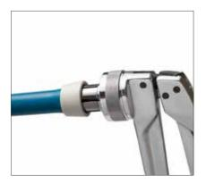
**3.** Using pipe expander, expand ring fully. Repeat expansions, rotating expander 1/8-turn between expansions.
