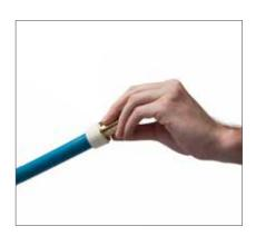
**4.** Insert fitting into expanded pipe and ring. Assure proper expansion so that fitting is touching pipe and ring. Hold fitting in place until pipe/ring memory constrict annularly around the fitting.
