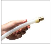
5. The installation is complete with a visibly secure connection. Remove defective connections. Test completed joint.
