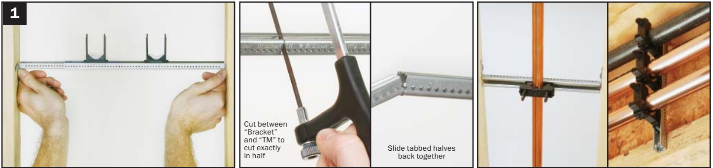
1 Bend tabs and expand bracket to fit opening. Fits 14"-24" openings.
