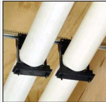
Large Pipe: use TouchDown II clamps for pipe up to 2".
